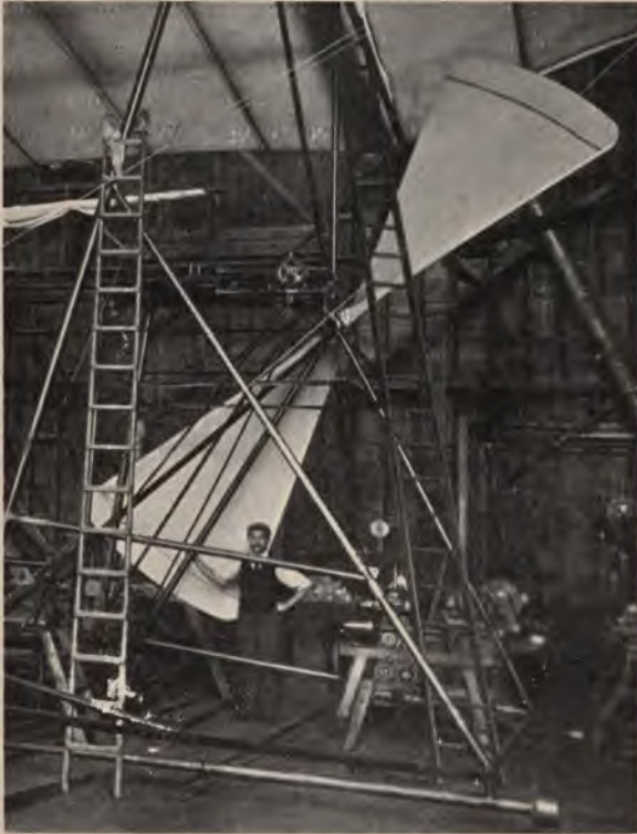
Fig. 89.—One of the large screws being hoisted into position. Its size may be judged by comparison with the man.
